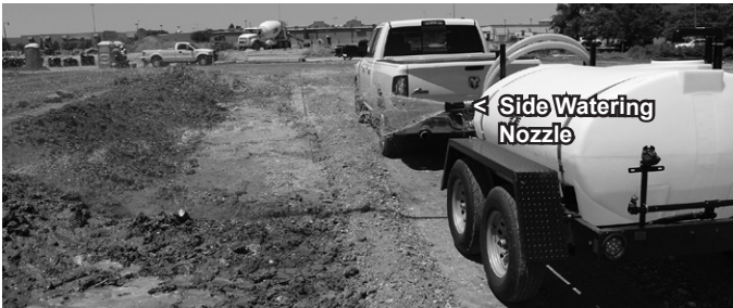
Figure B12 Side Watering Nozzle
