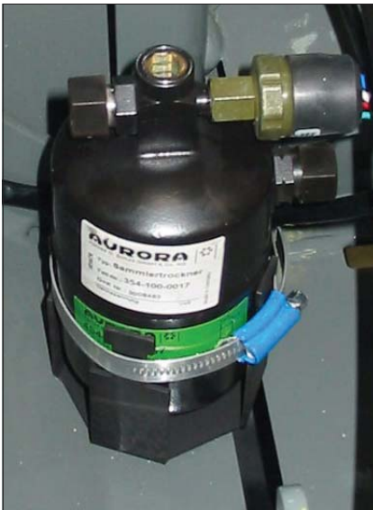
Fig. 2: Dehumidifier with pressure switch
