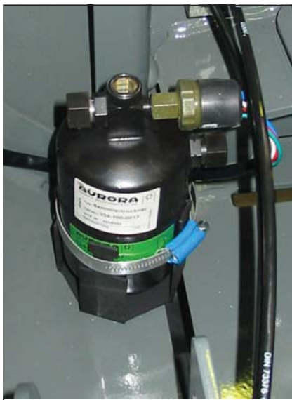
Fig. 2: Dehumidifier with pressure switch
